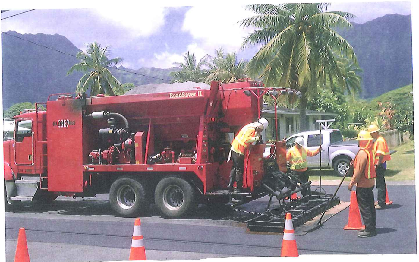
Slurry seal truck at work
