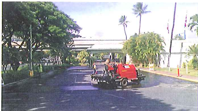
Sealcoat being applied to pavement
